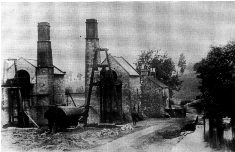
The Pumping Engines at Dunkerton
